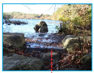
The spillway dam of Wash Pond provides a hydraulic control of pond level. However, the pond depth just east of the dam is shallow. The natural pond base here and the low gradient drop to the Hale House ram pump location provide evidence that this low structure is designed only to help maintain p o n d level during dry tiples.
